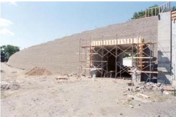
The stiff requirements for the roadway made the design of the off ramp a challenge. The retaining wall design needed to meet the specifications of the American Association of State Highway and Transportation Officials (AASHTO). The city requires that all retaining walls with state roads above them must be designed according to these standards. AASHTO design specifications require that the minimum geogrid reinforcement lengths must be 70% of the wall height.
