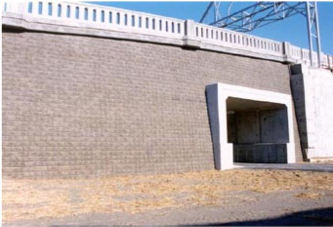
The construction of the Herrick Street Bridge needed to be very well thought-out. The surveying team spent many hours laying out the placement of the walls and accounting for the block setback. This was especially critical since the design required the two walls to have 31 feet (9.45 m) of spacing between them at the top.
